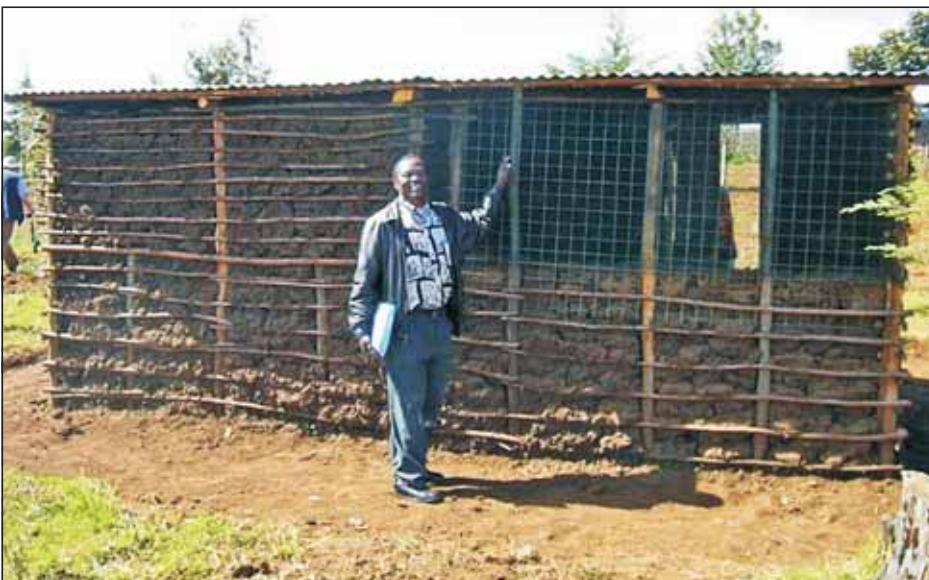
A new, bee-proof, processing hut, built mainly using local materials
